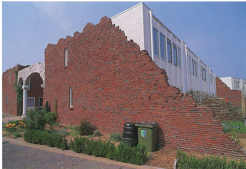
Tendencies of facadism in The Netherlands. Leo Heijdenrijk. ‘Ruins’, social housing, Amersfoort, 1992
