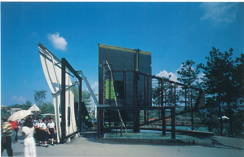
Exhibition pavilion for the 1990 Osaka Expo of Gardens and Greenery
