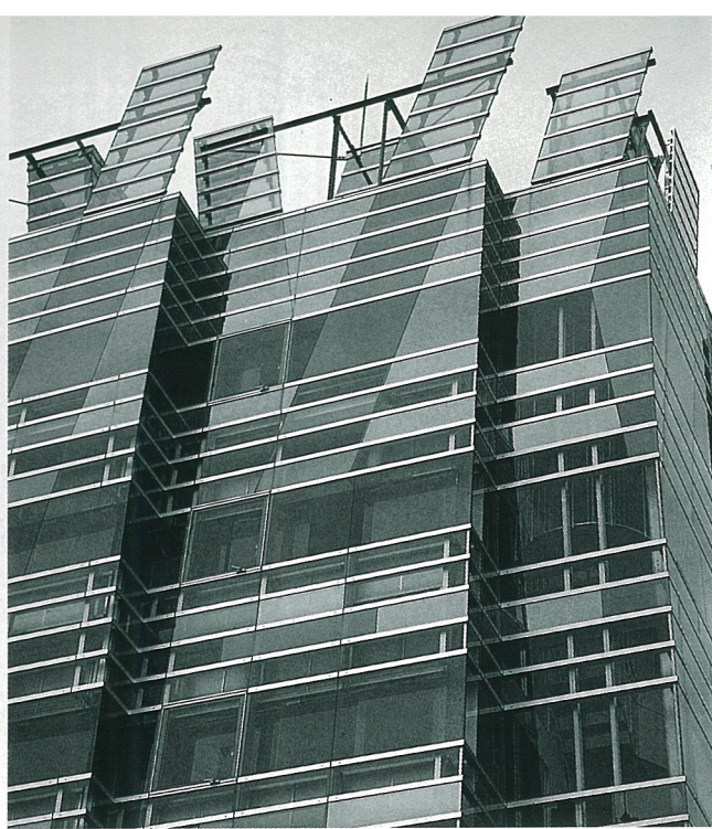
STM House, Tokyo, 1991
