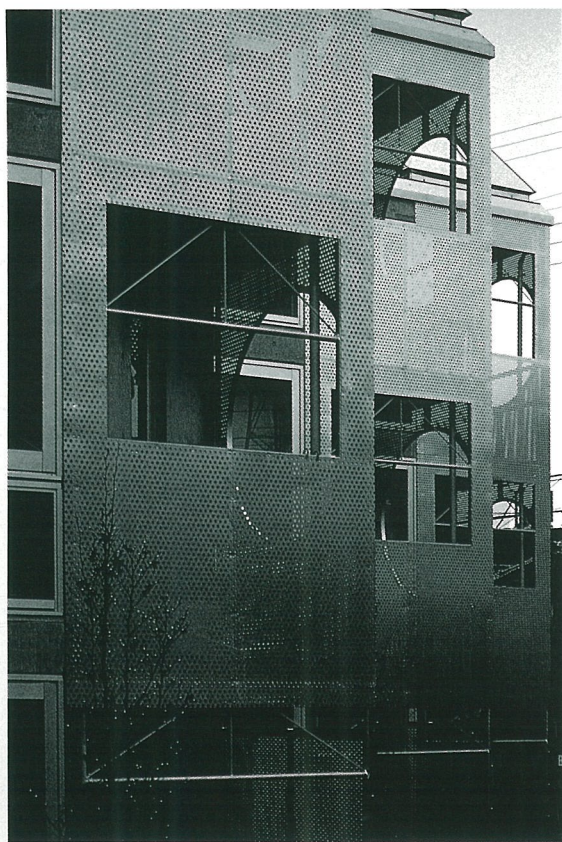
NC House, Tokyo, 1983
